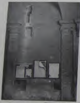
Fig. 115. S. Sebastiano. Splice of masonry showing evidence of posthumous removal of corner pier.
